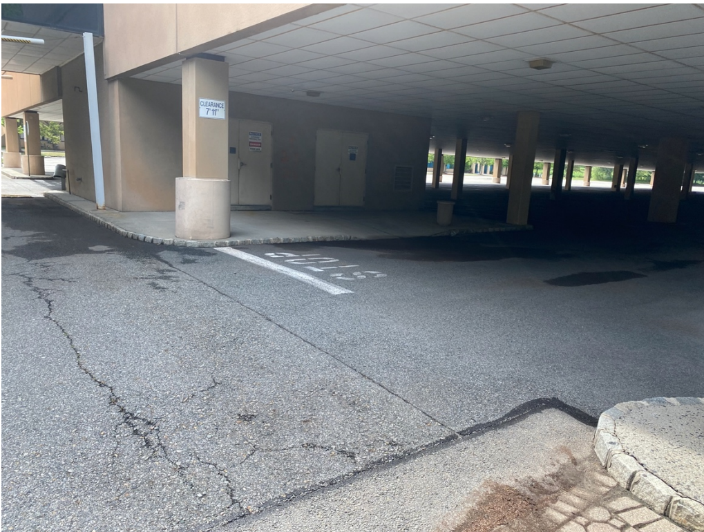
Figure 14: Lack of pedestrian facilities
