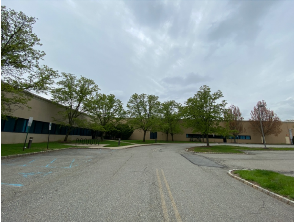
Figure 16: Lack of crosswalk, another non-ADA compliant sidewalk ramp adjacent to ADA spaces; faded circulation striping
