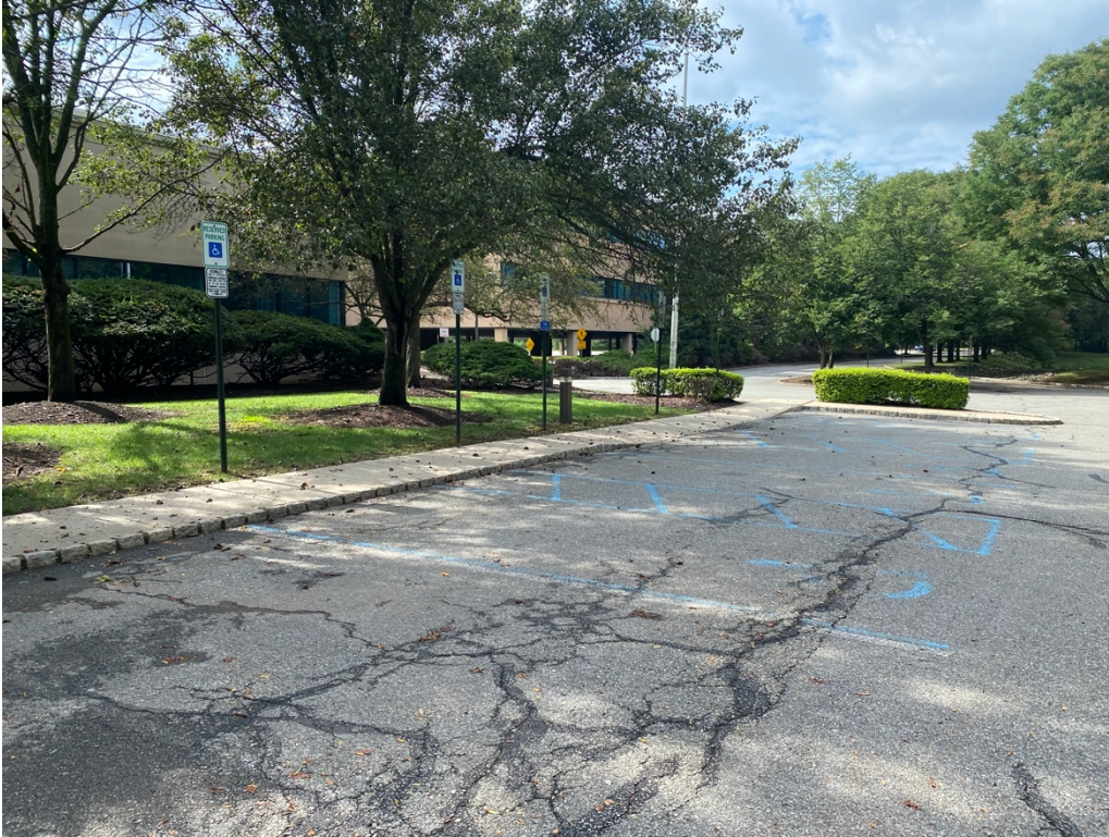
Figure 21: ADA accessible parking area
