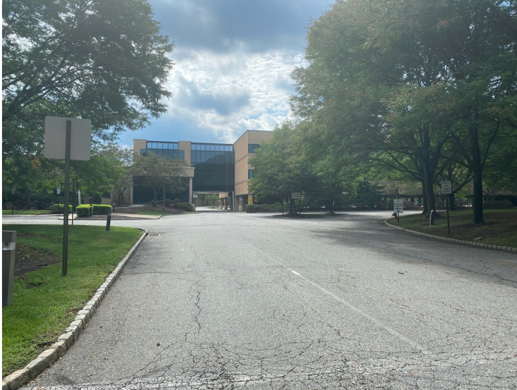
Figure 32: View of the Site from only curb cut
