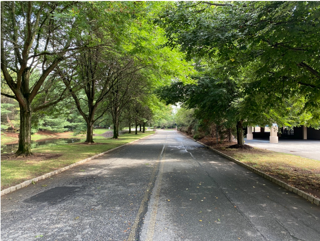
Figure 4: Patched access road with faded striping
