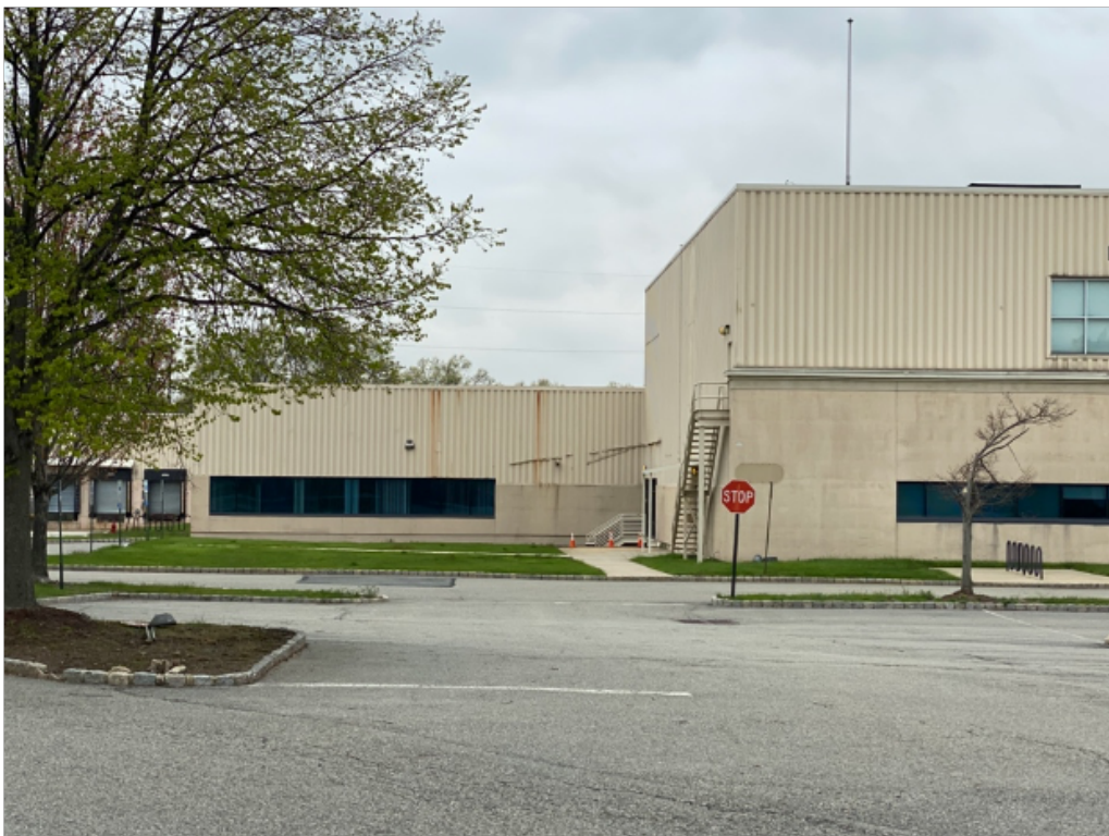
Figure 10: Damage to foundation and façade
