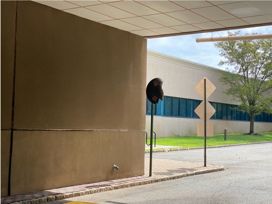
Figure 1: Broken safety mirror
