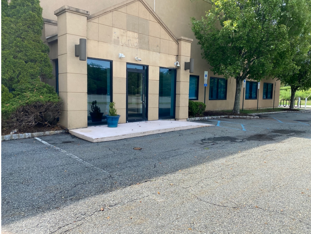
Figure 23: A traffic conflict with adjacent ADA accessible parking spaces
