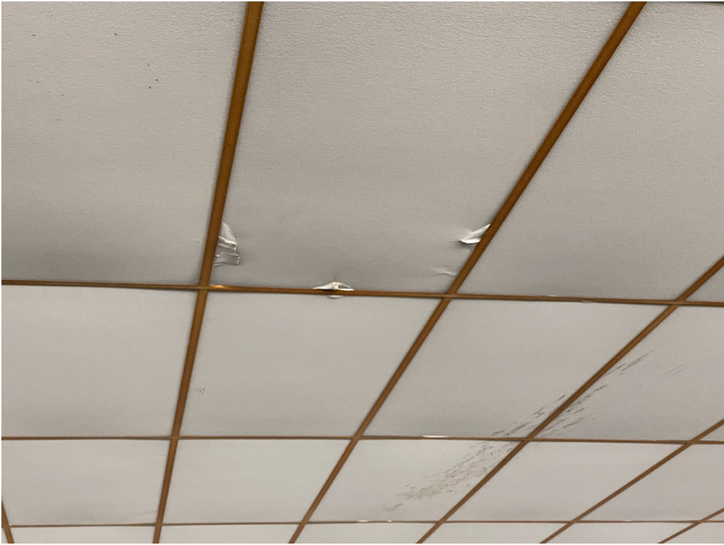
Figure 12: Water infiltration (3)
