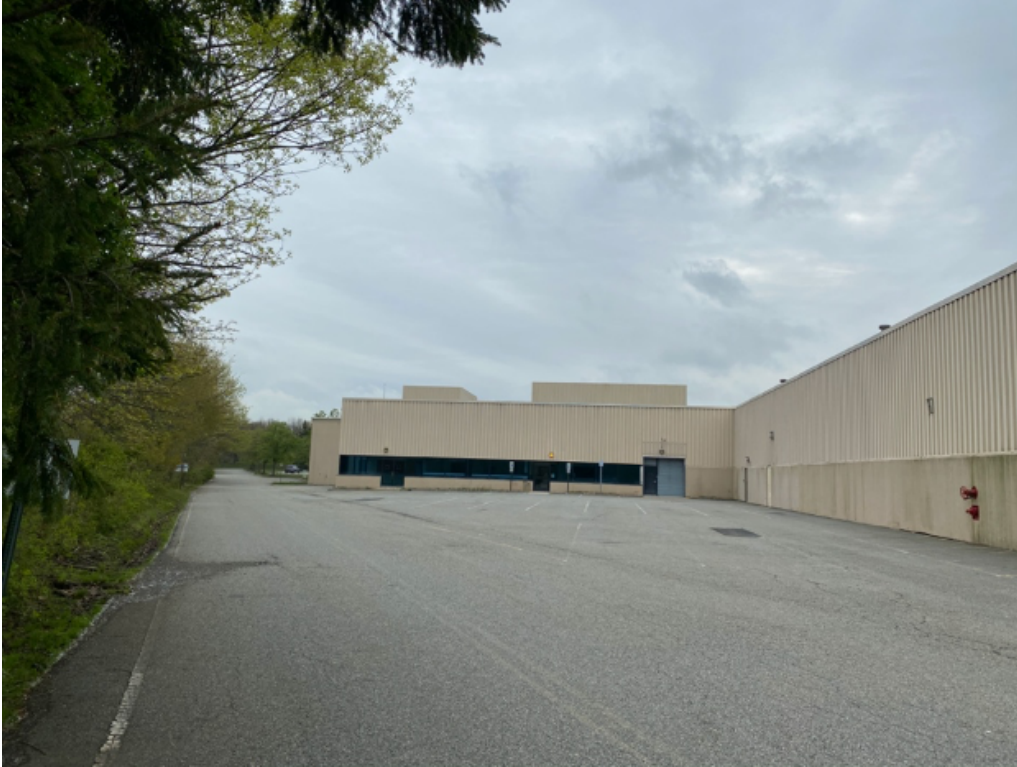
Figure 40: Completely impervious area located on the site
