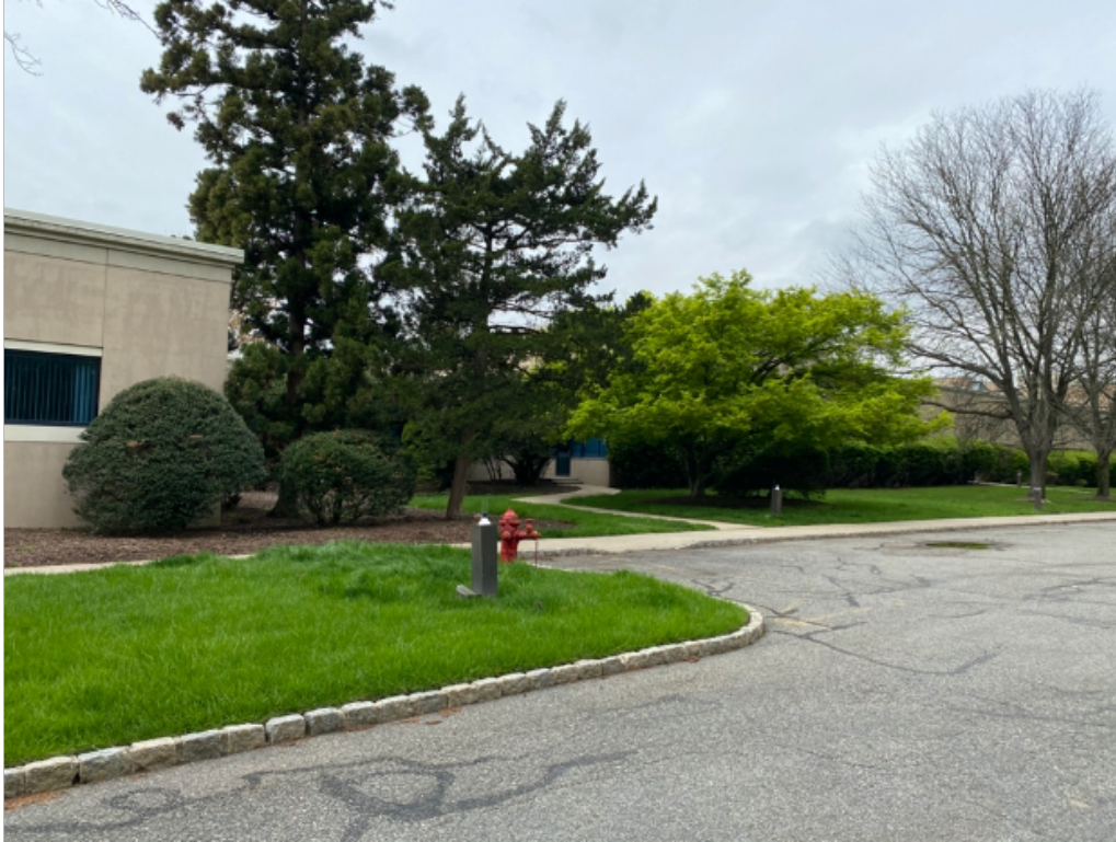
Figure 13: One of the broken pedestrian safety lights
