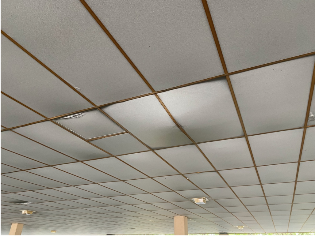
Figure 11: Water infiltration (2)
