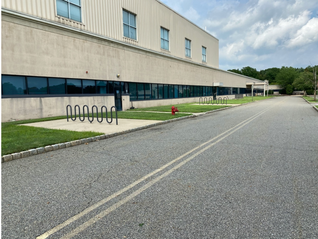
Figure 25: Non-ADA-compliant pedestrian controls
