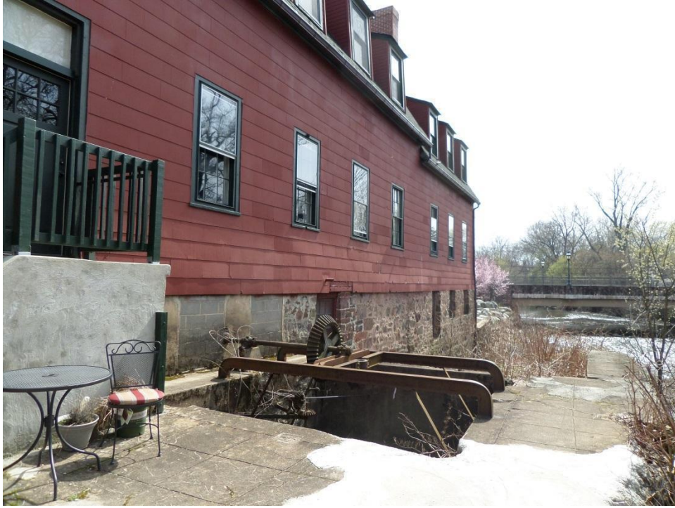
Photograph 5: View facing south-southwest showing concrete cover and well above the millrace.
