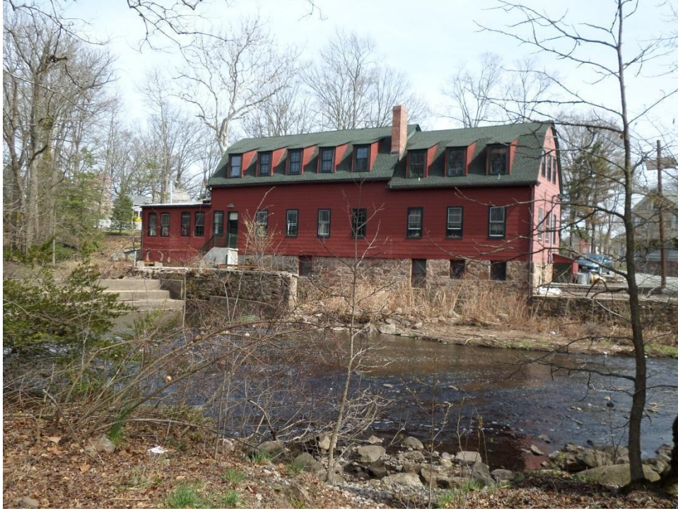
Photograph 3: View facing east-northeast showing the northwest elevation of Droschers Mill.
