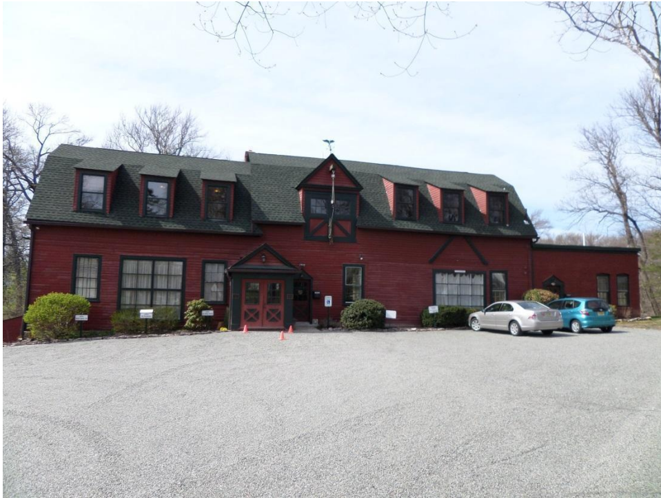
Photograph 1: View facing northwest showing the southeast elevation of Droschers Mill.
