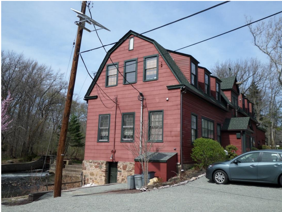
Photograph 4: View facing north showing the southwest elevation of Droschers Mill.
