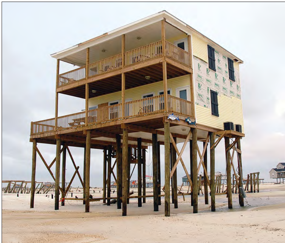
Figure 3-10. Home elevated on piles.
