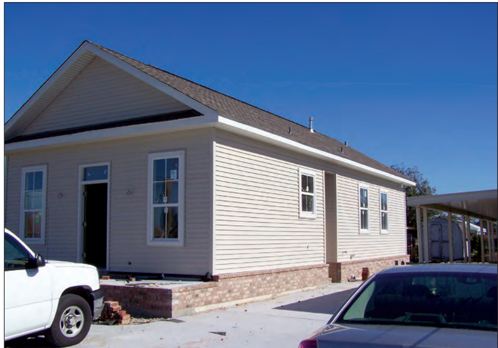
Figure 6-9. Typical mitigation reconstruction project.
