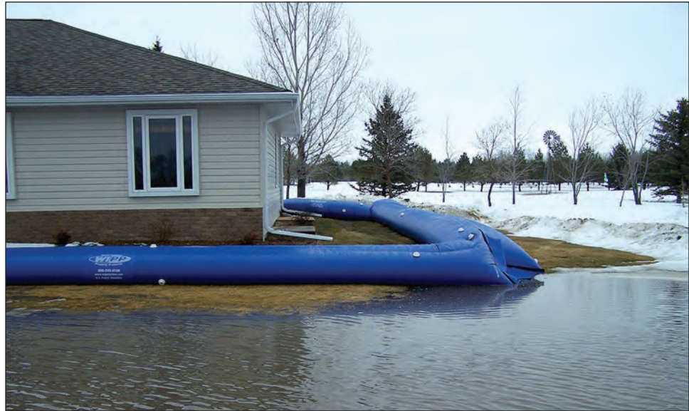
Figure 8-4. Two-foot-high water-filled temporary barrier protecting a residence from flooding (2010 – Courtesy of Hydrological Solutions, Inc.).
