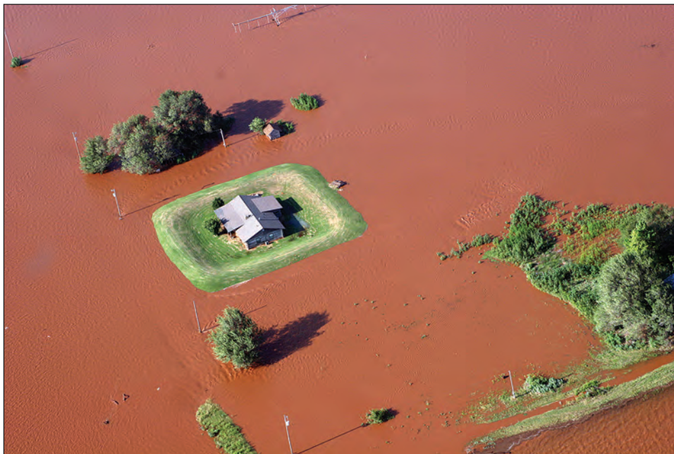
Figure 3-18. A home protected by a levee.
