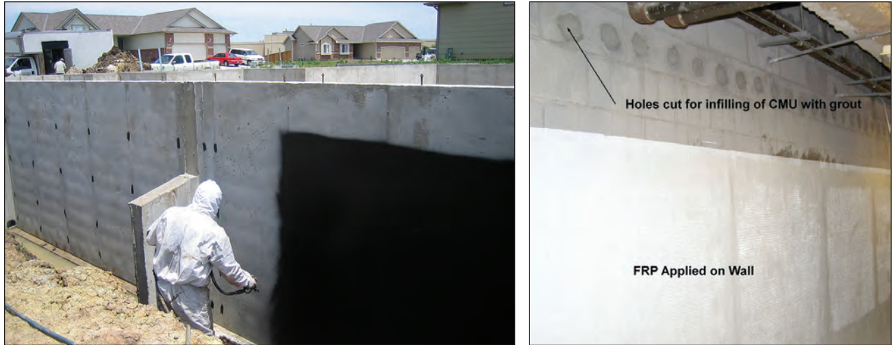
Figure 7-5. Example of an exterior application of a spray-applied asphalt membrane (left – courtesy of GMX, inc.) and an interior application of a fiber reinforced polymer wrap (right).
