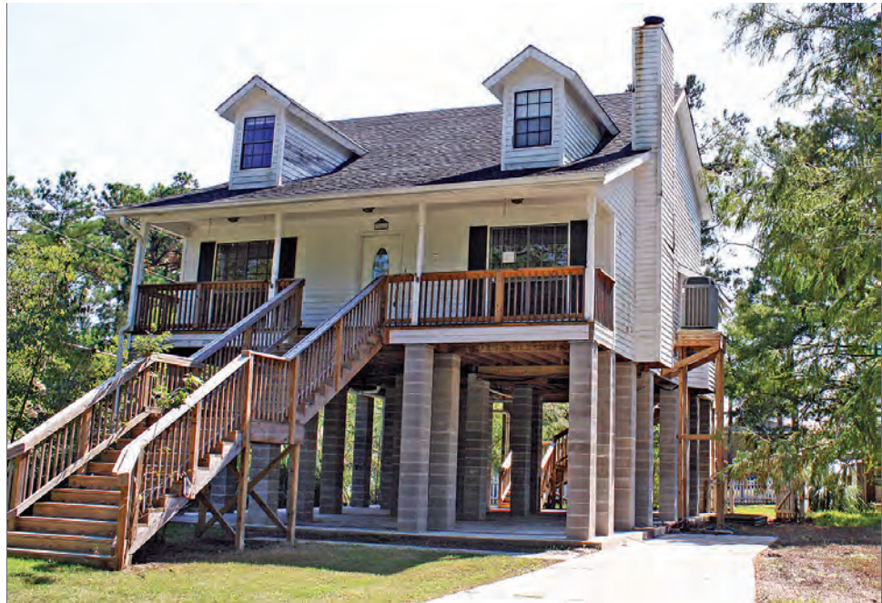
Figure 5-8. House in Zone A was detached from its slab foundation (which remains) and elevated on masonry piers. The floor system is supported by new wood joists (Mandeville, LA).
