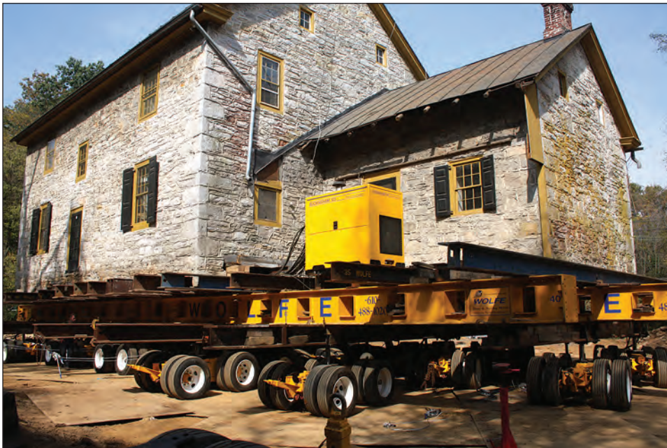
Figure 6-6. Trailer wheel sets are placed beneath the lifting beams (photo courtesy of Wolfe House Movers).
