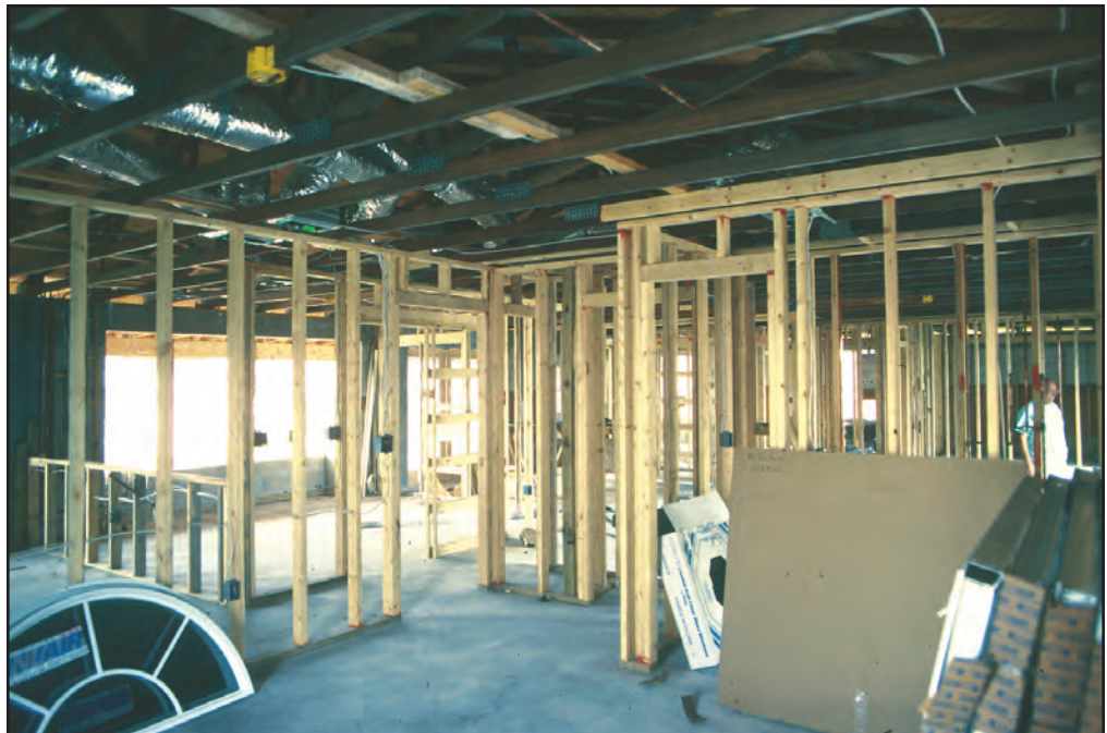
Figure 30 Interior partition walls and utilities are added.
