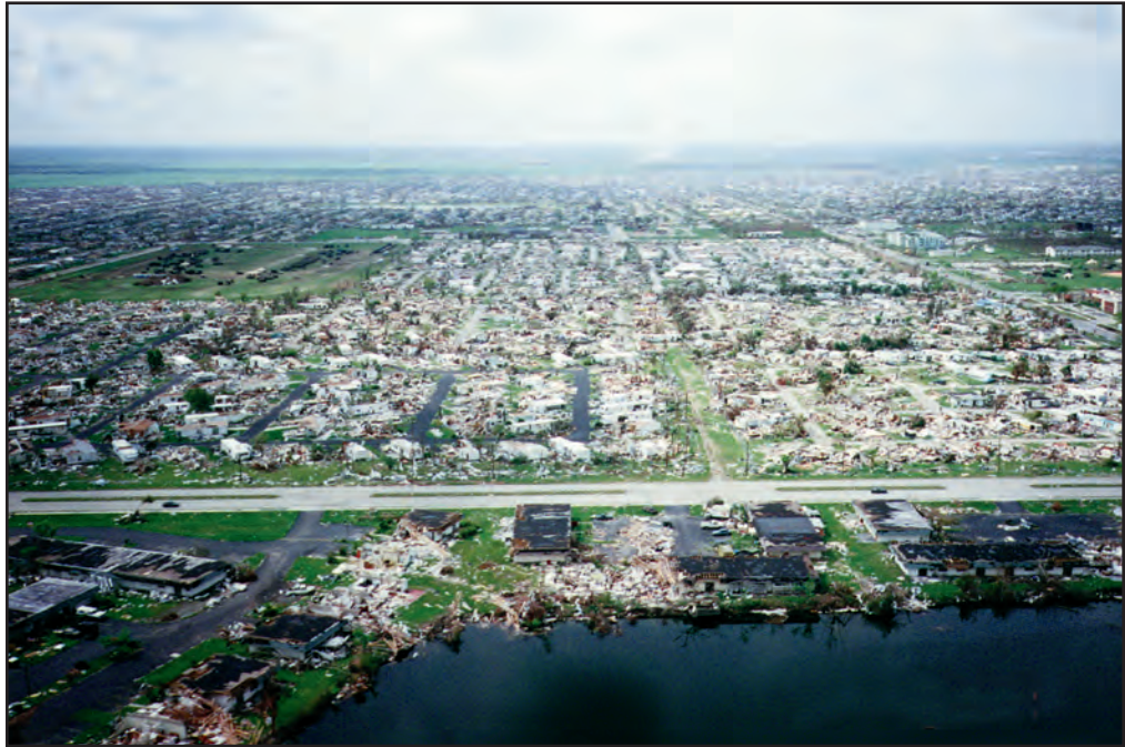
Figure 2 Damage to houses and other buildings was severe.
