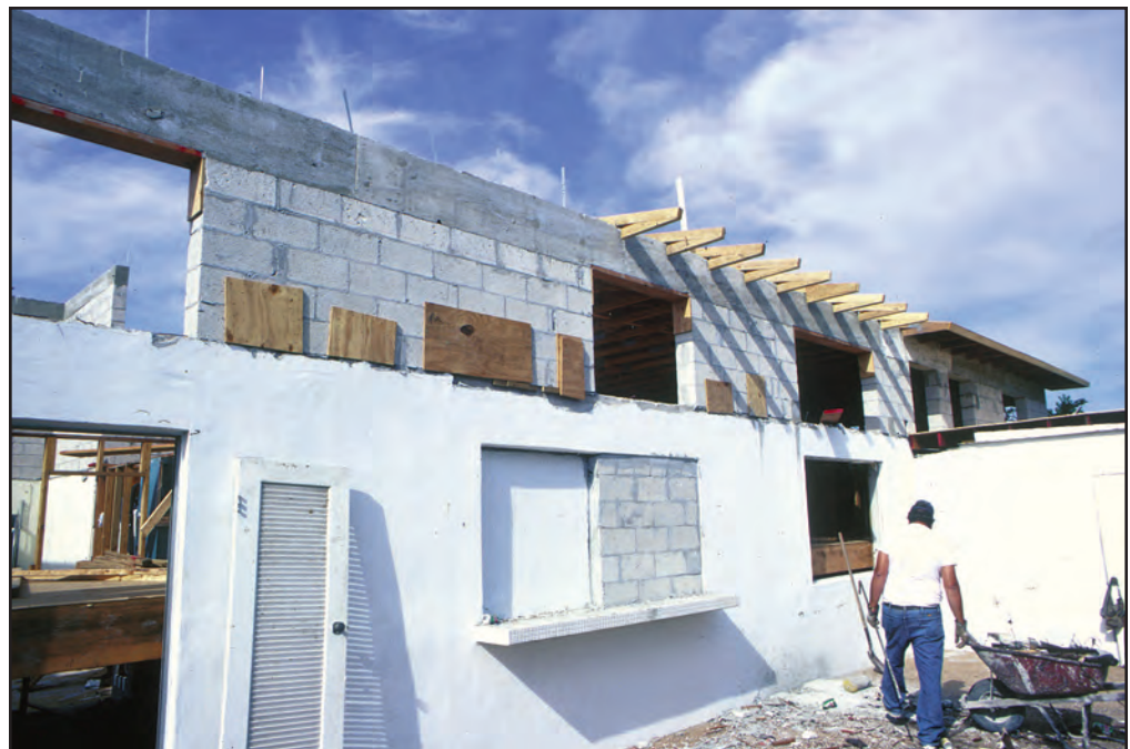
Figure 67 The extended first-story walls.
