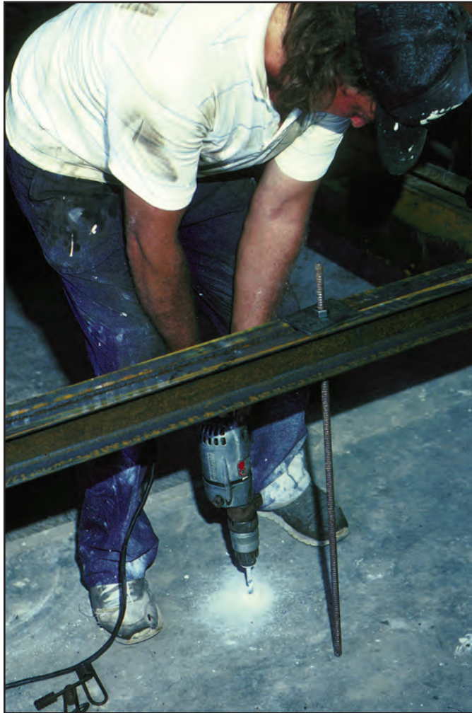
Figure 77 ... install anchors ...
